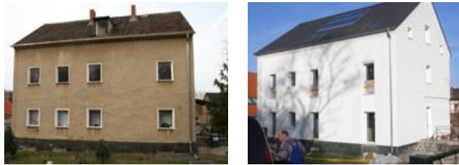
Figure 8: Old and New Facade Views of B-5, Brandenburg/ Germany (Passive House Database, 2023).
