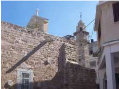
Figure 3: Saint Porphyrius church and Kateb Al Wilaya Mosque share the same wall.
