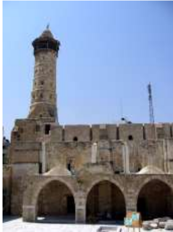
Figure 10: North elevation of the prayer hall of GOM.
