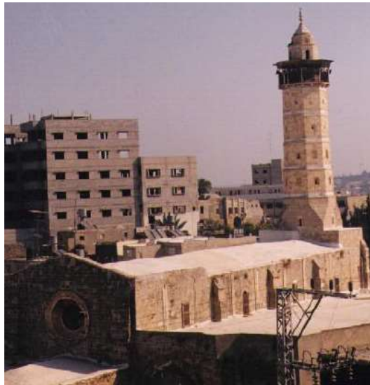
Figure 4: View of the GOM.
