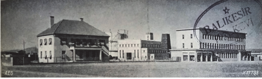
Figure 4: Ankara Power Plant (Işıkpınar 1932)
